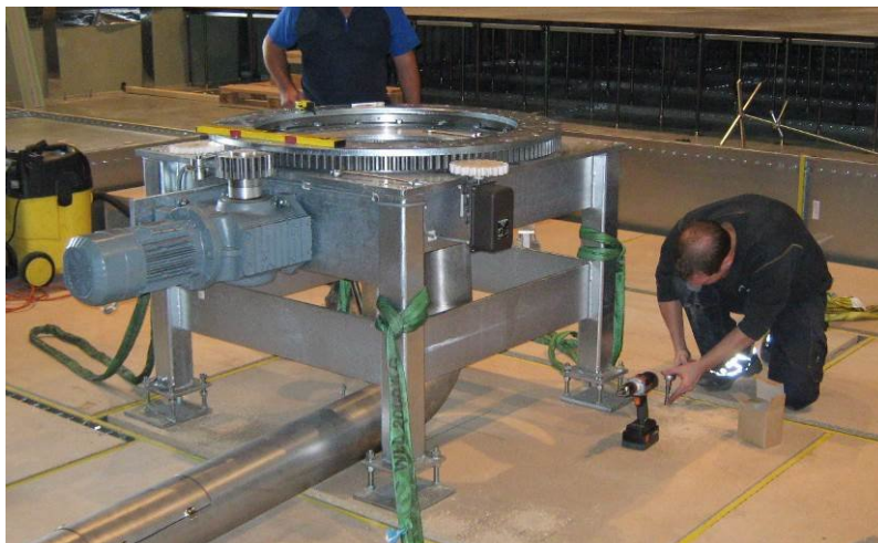
Fig.: Drive unit assembly of turntable
