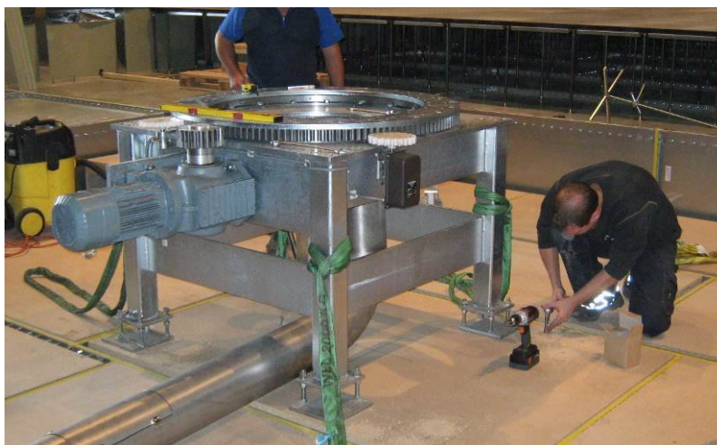
Fig.: Drive unit assembly of turntable
